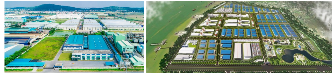
Dai Dong Hoan Son IP in Bac Ninh province Perspective drawing of Nam Tan Tap IP project in Long An province
