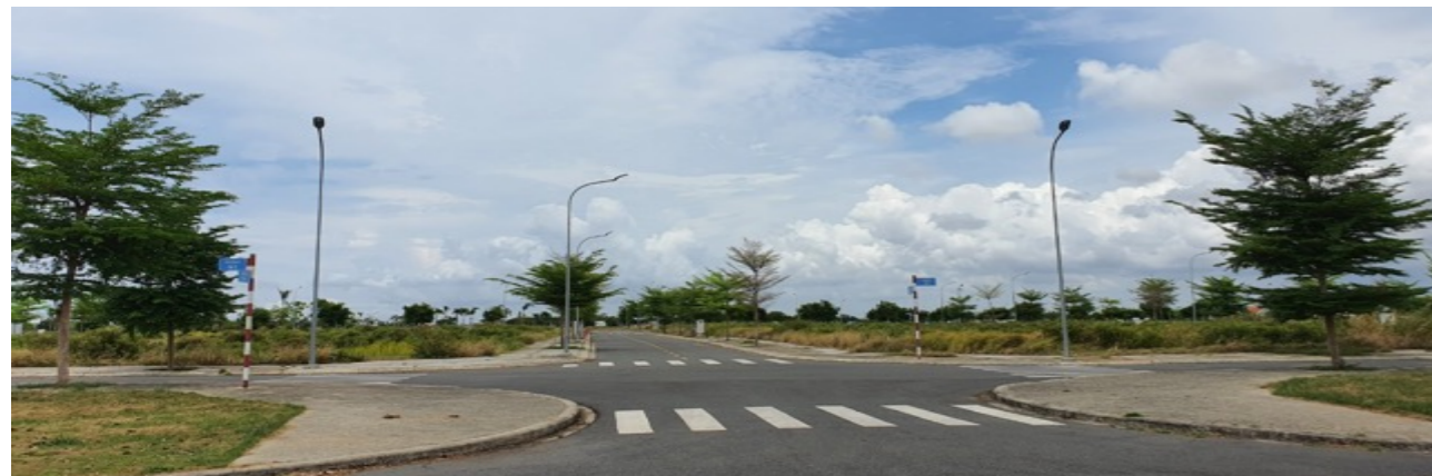
Infrastructure in Long An IC and RA
