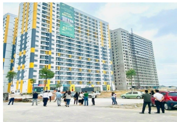
SH project in Nenh town - Bac Giang Phase 1 is putting into use in 2024
